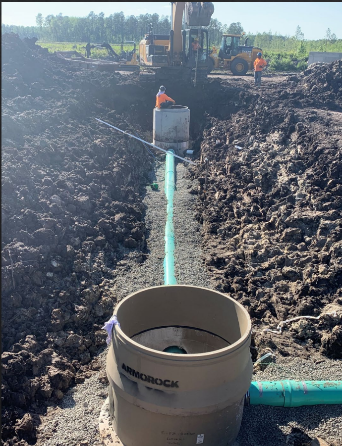
ILP Gravity Sewer & Polymer Receiving Manhole
