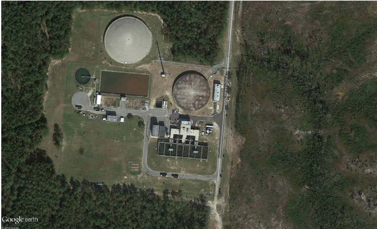
Figure 1-2 Aerial View of Northwest WTP
