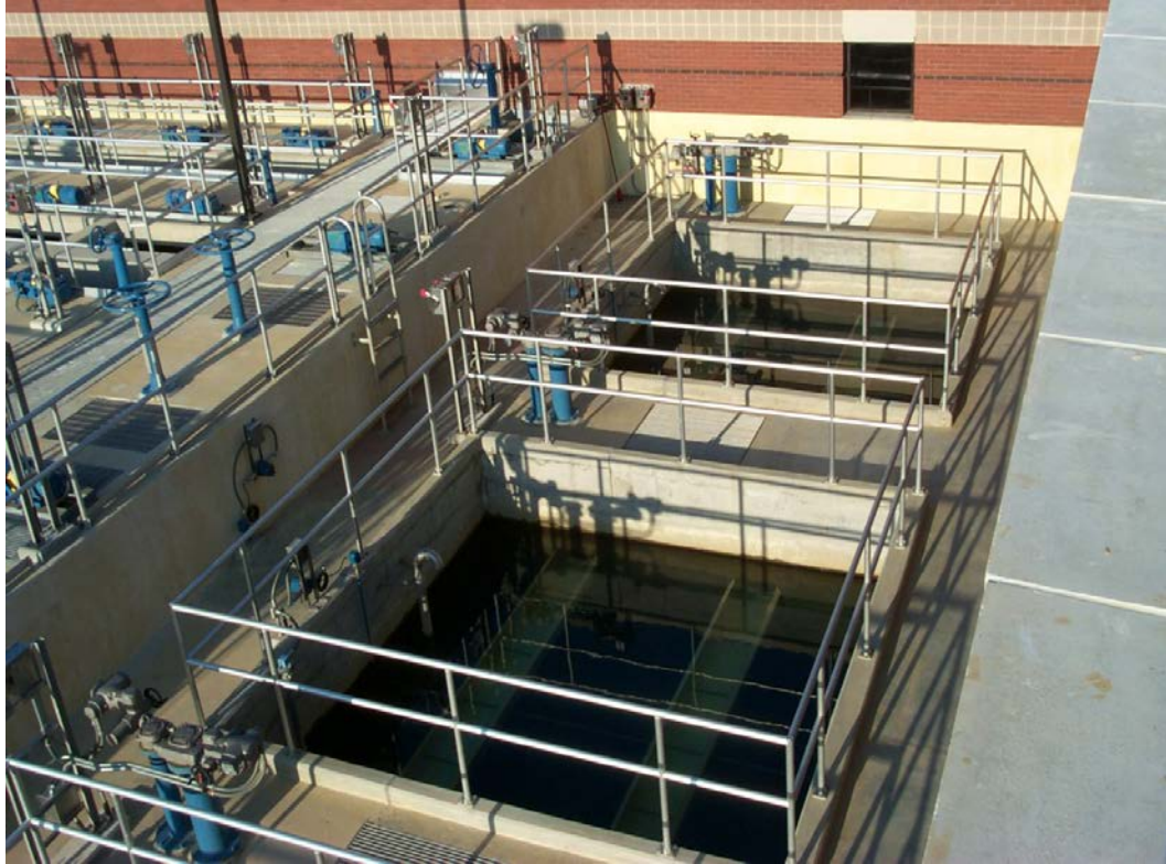
Figure 3-2 GAC Gravity Filter
