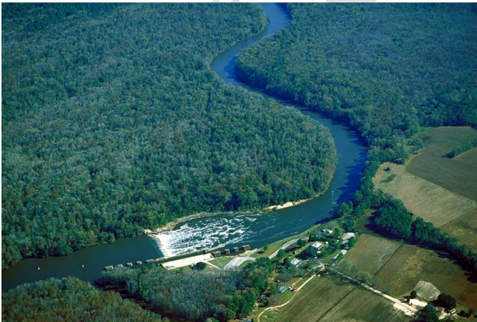
Figure 1-1 Lock and Dam No. 1 on the Cape Fear River
