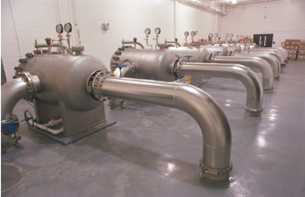
Figure 5-3 Horizontal Cartridge Filter
