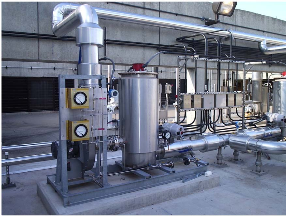
Figure 6-7 Ozone Offgas Blower and Destruct Unit Skid at Fairfax Water Corbalis WTP
