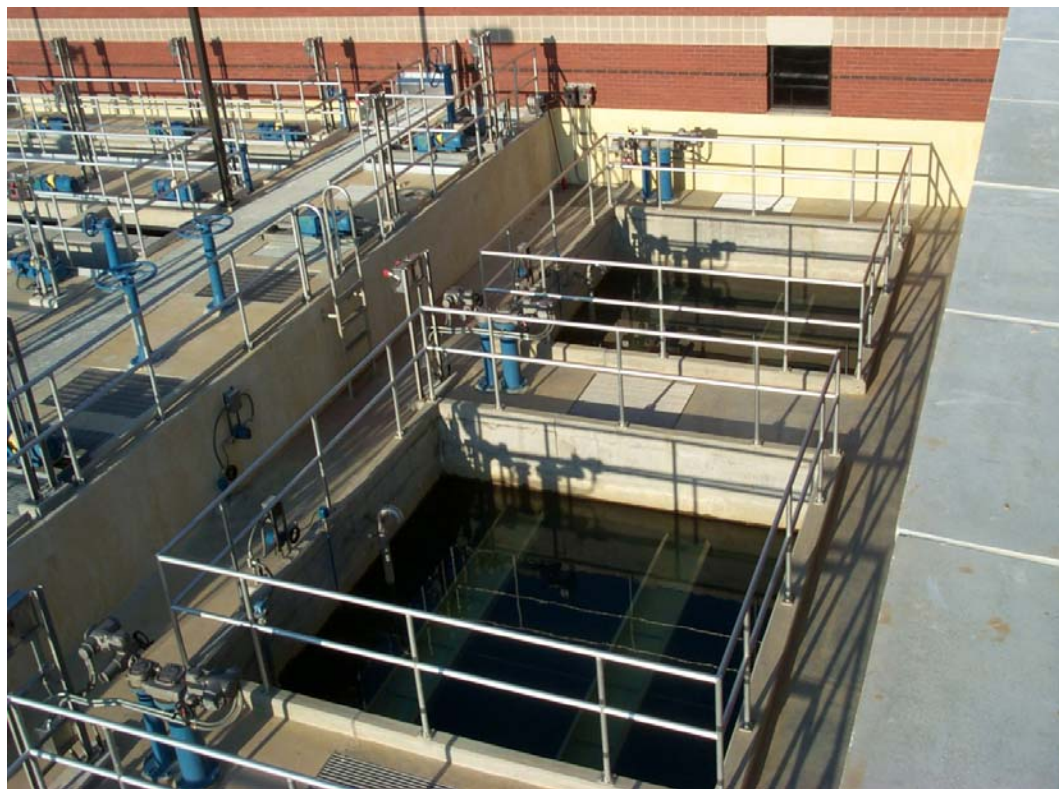
Figure 3-2 GAC Gravity Filter
