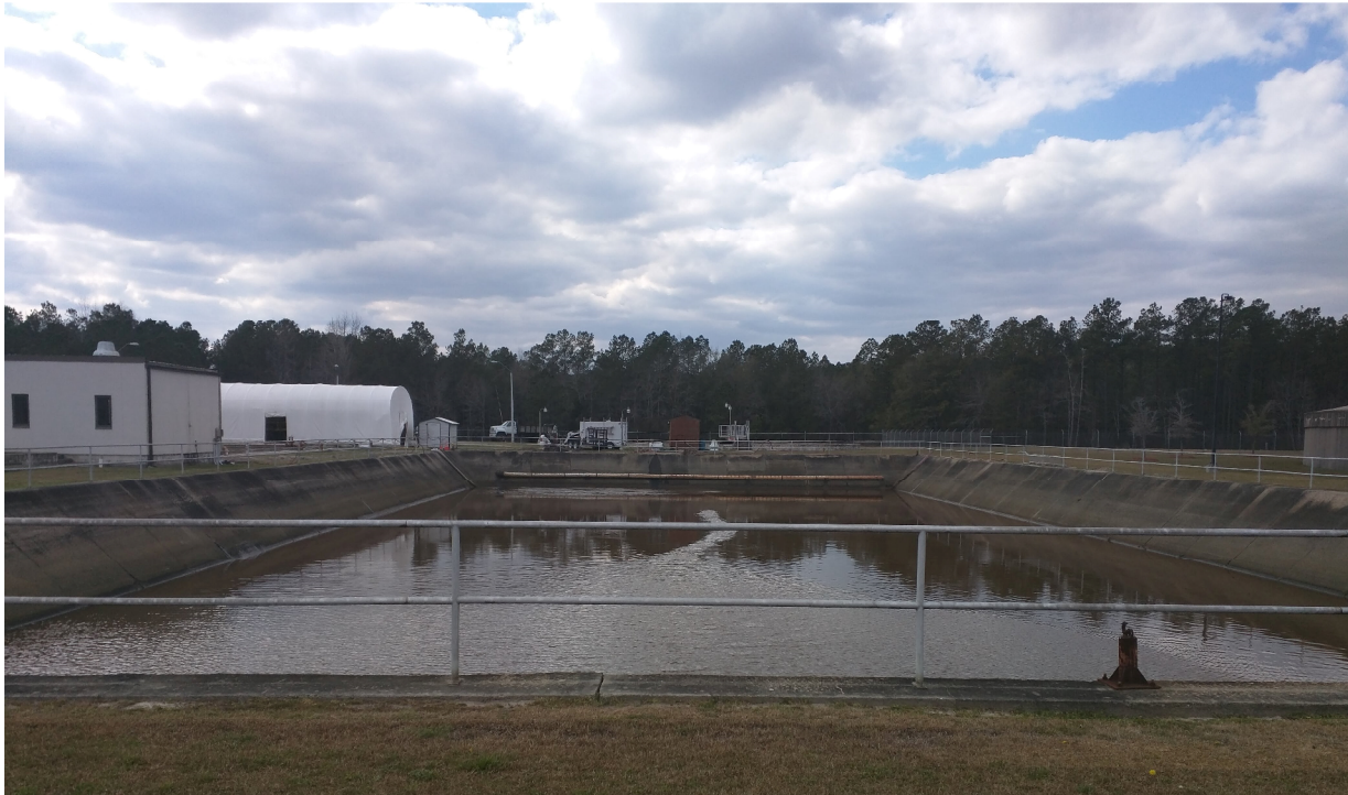
Figure 8-2 Residuals Equalization Basin
