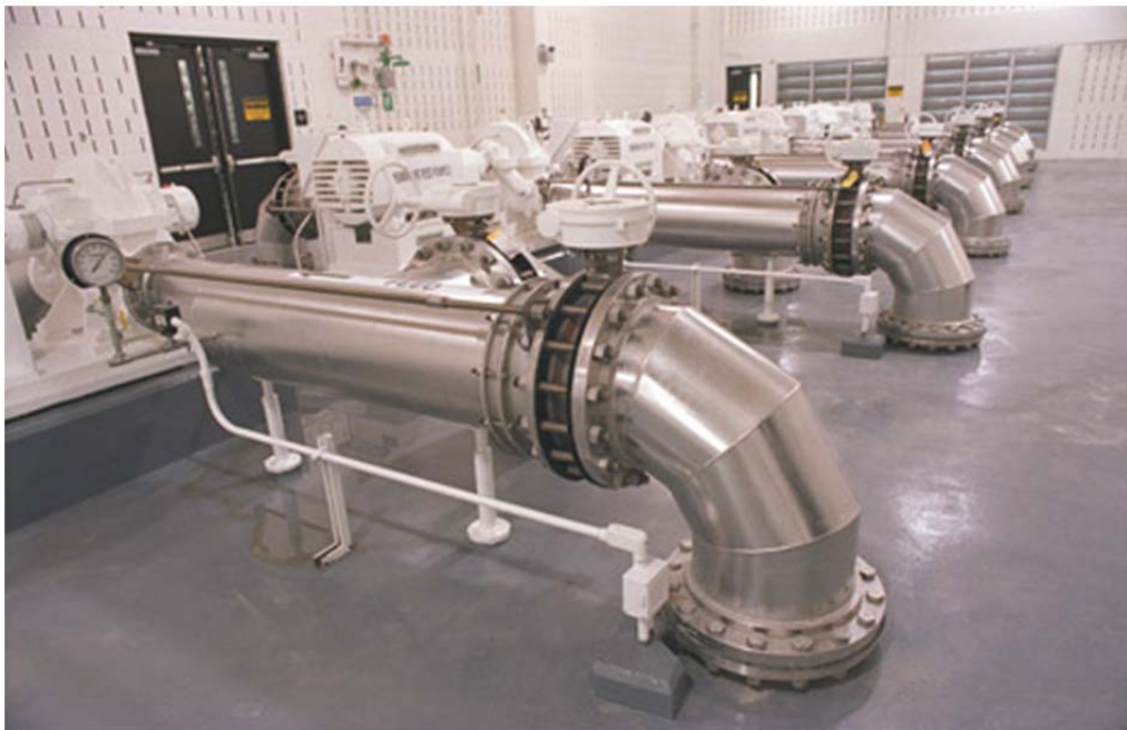
Figure 5-4 Horizontal Spilt Case RO Feed Pumps
