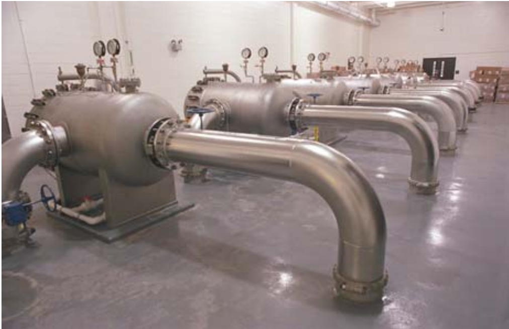
Figure 5-3 Horizontal Cartridge Filter
