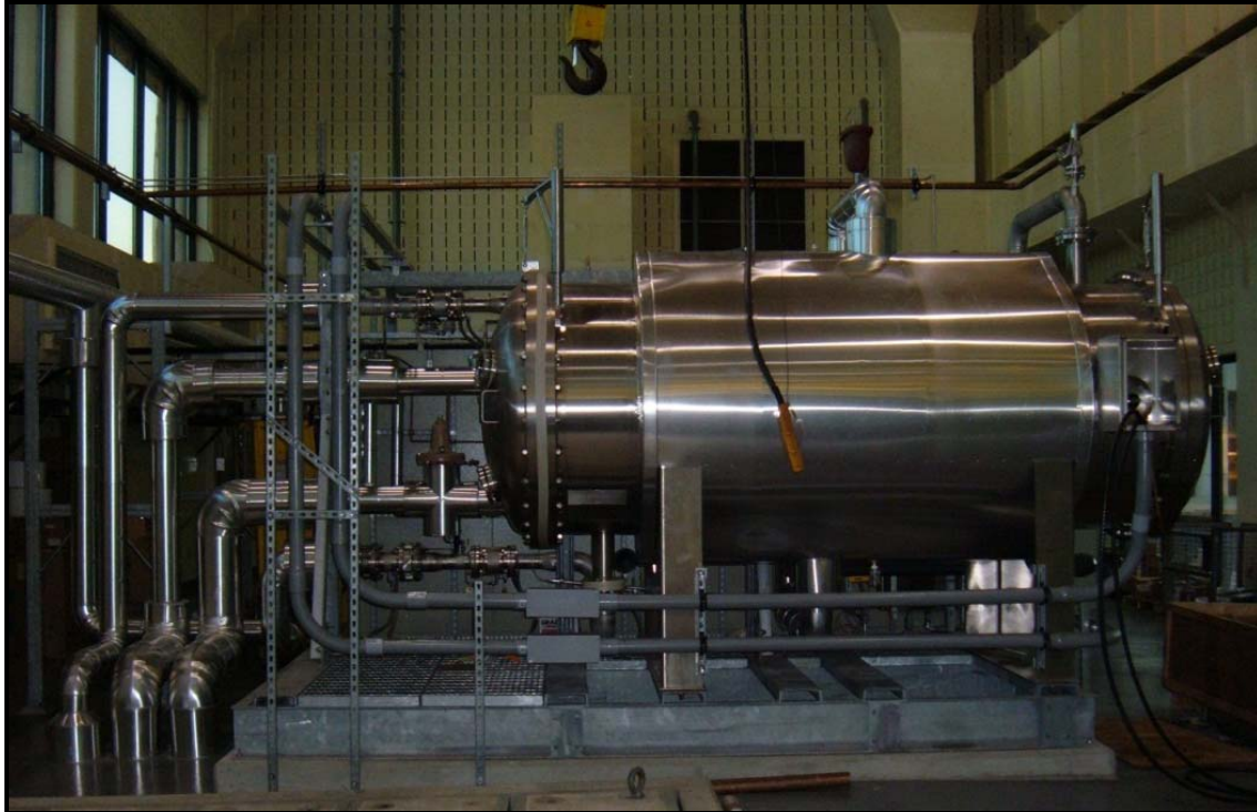
Figure 6-5 Ozone Generators at Corbalis WTP
