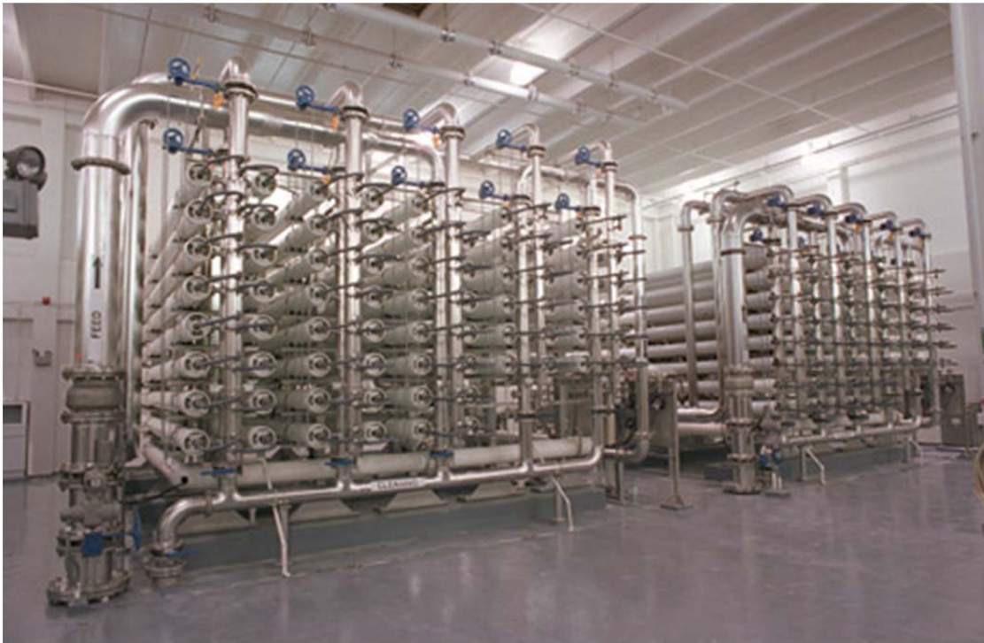
Figure 5-5 Two-Stage RO Membrane Skids Using Standard 8-Inch Diameter Pressure Vessels
