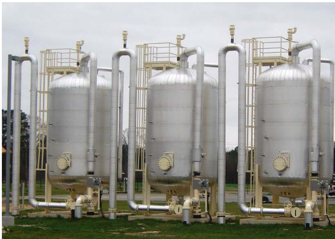
Figure 3-3 GAC Pressure Contactors
