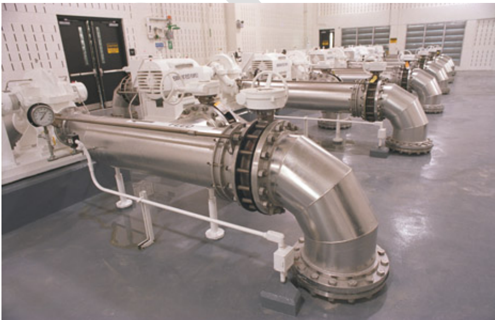
Figure 5-4 Horizontal Split Case RO Feed Pumps
