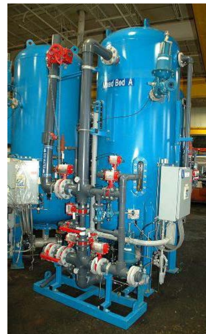
Figure 4-3 Ion Exchange Pressure Vessel
