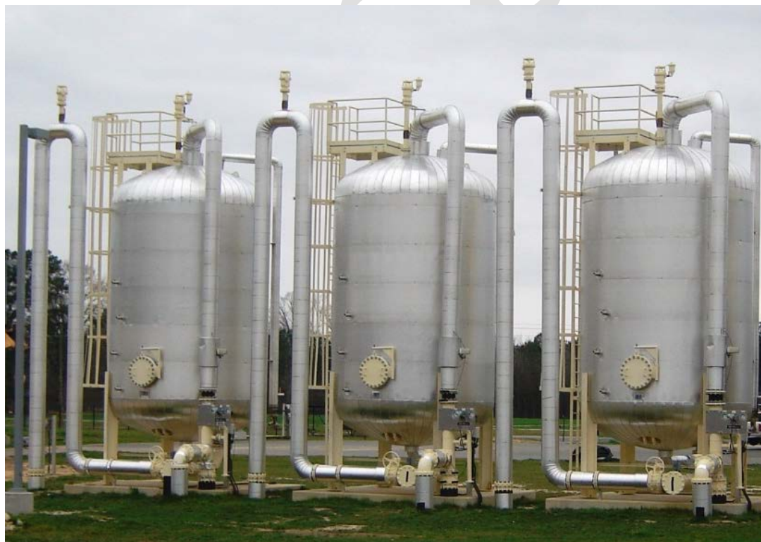
Figure 3-3 GAC Pressure Contactors
