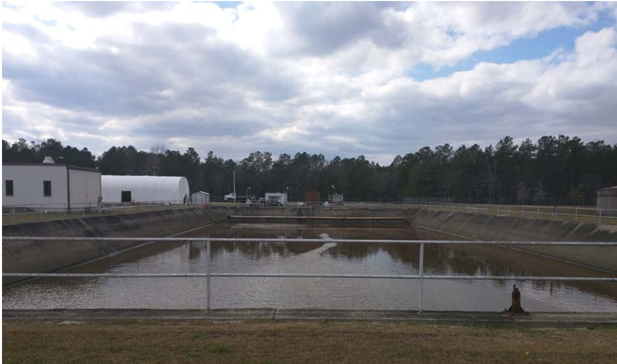
Figure 8-2 Residuals Equalization Basin
