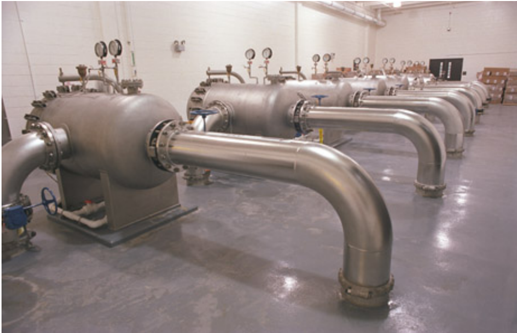
Figure 5-3 Horizontal Cartridge Filter
