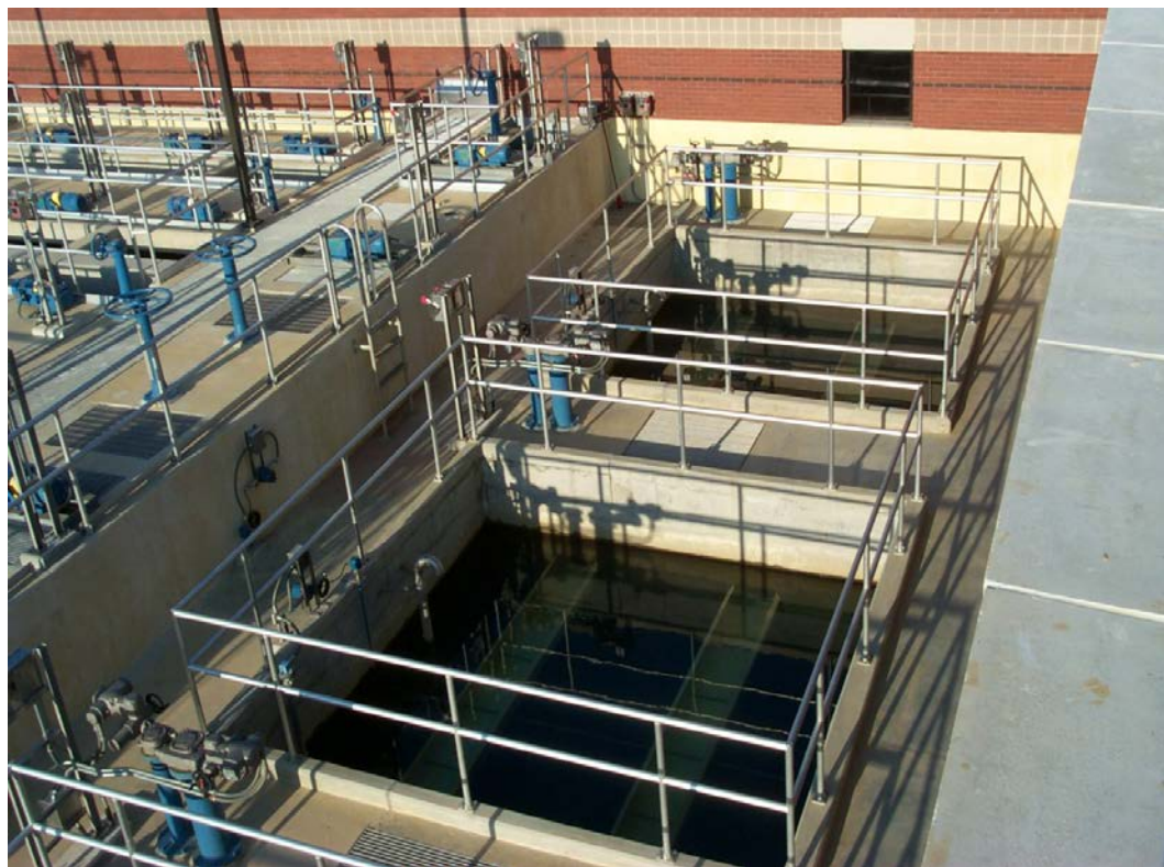
Figure 3-2 GAC Gravity Filter
