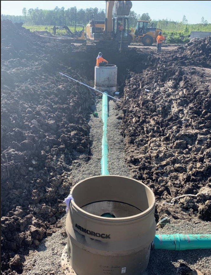
ILP Gravity Sewer & Polymer Receiving Manhole
